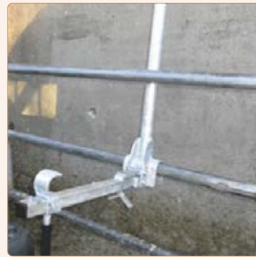
BO-STEEL ANTI-BACKING BAR CONECN011 Removable Anti-Backing bar.
